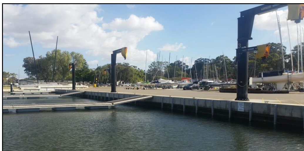
South of Perth Crane, Hardstand and Floating Collector Jetties
