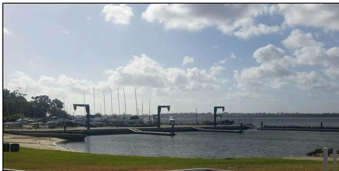
Crane and Hardstand facilities viewed from the SoPYC Clubhouse
